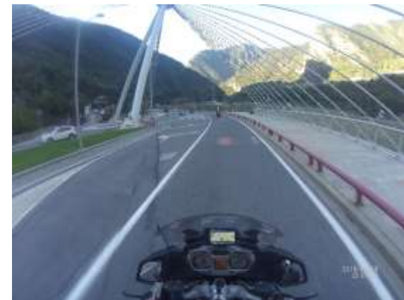
Cable-stayed road-bridge on the N145 after leaving Andorra.
