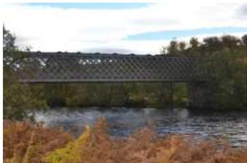
A couple of 100m away is an impressive, riveted, lattice girder bridge, made by McFarlanes of Dundee in 1863 and which now, is another category A listed structure. Walkers and cyclists still cross this bridge because it forms part of the Speyside Way.
